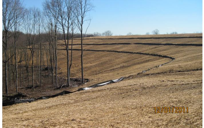
Recontoured and seeded hillside after removal of gob and spoil piles
