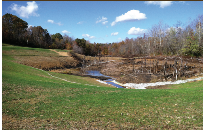
Lake Morrow post construction Photo by Sarah Landers
