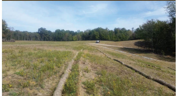
Surface reclamation complete with regrading, seeding, and limestone channel Photo by Amy Mackey
