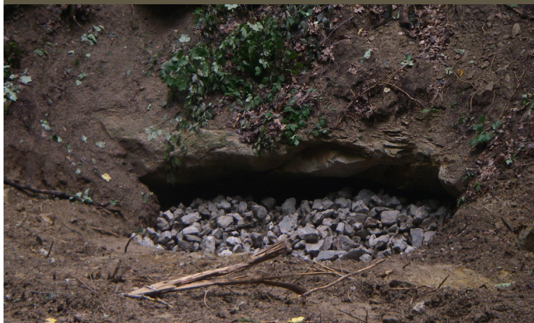
Lost Run Subsidence (site CDE) in-progress closure
