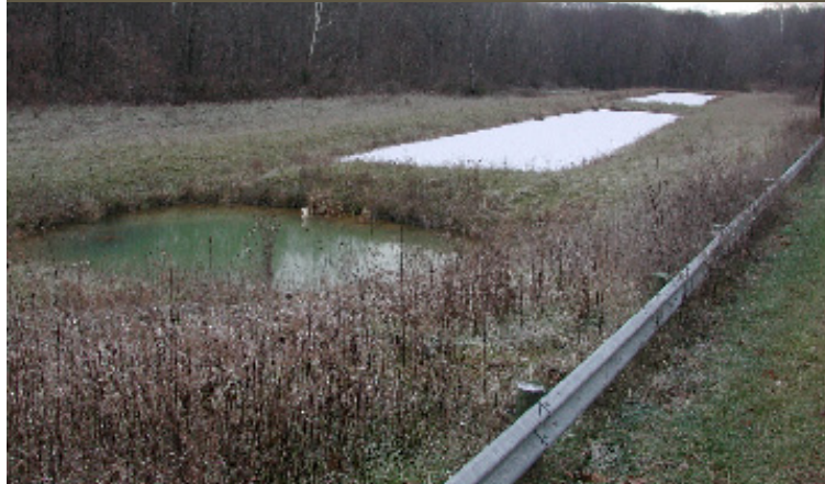
Successive Alkaline Producing System (SAPS), Photo by Ben McCament
