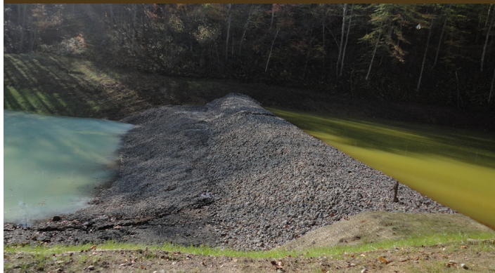
Coe Hollow Limestone Leach Berms (USFS) Photo by Monday Creek Restoration Project
