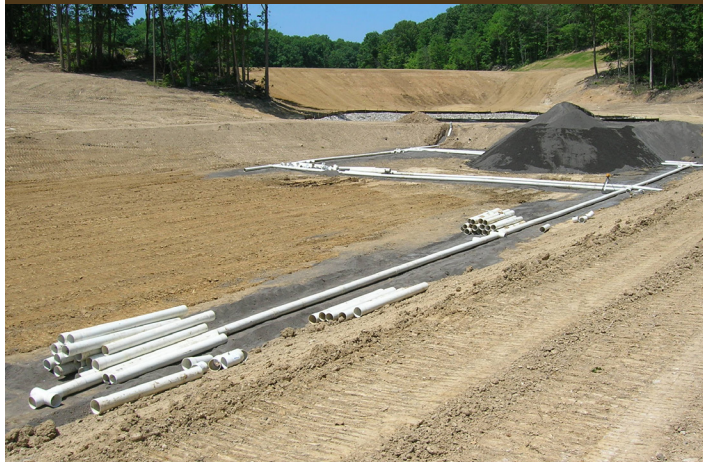
Steel slag bed downstream Lake Milton, Photo by Ian Hughes
