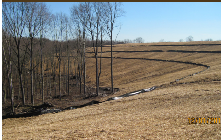
Recontoured and seeded hillside after removal of gob and spoil piles Photo by Amy Mackey
