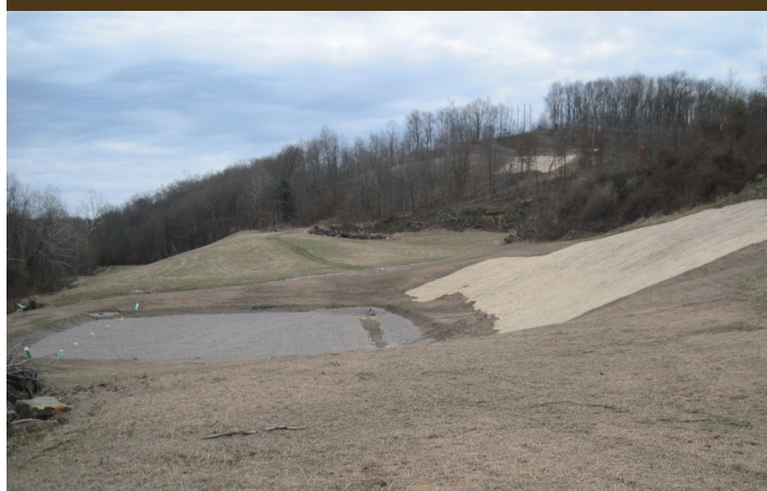
West Branch Headwaters limestone leach bed. Photographer: Michelle Shaw
