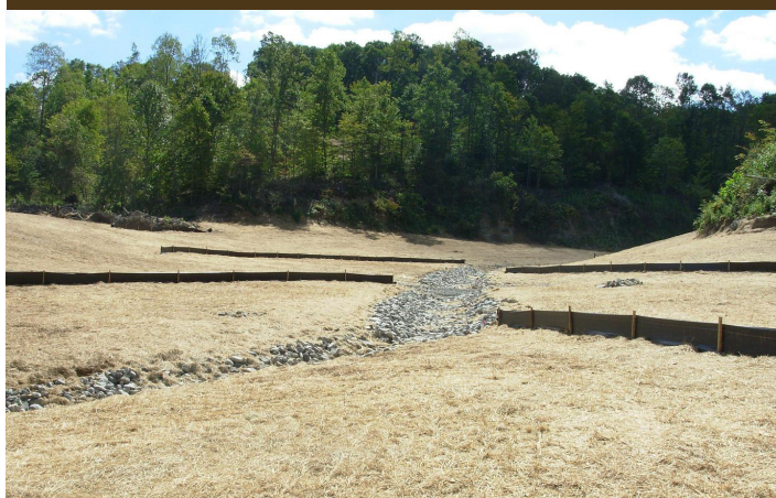
West Branch Sunday Creek Phase I post reclamation featuring a limestone channel. Photographer: Sunday Creek Watershed Group
