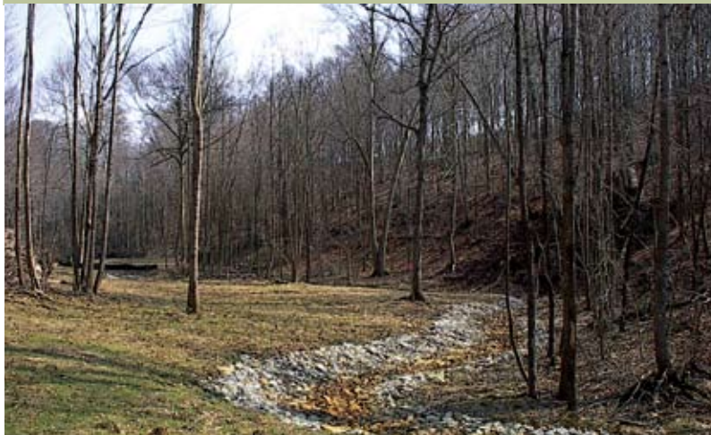
Lost Run Open Limestone Channel (1W5)
