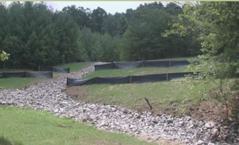
Regraded and resoiled gob pile
