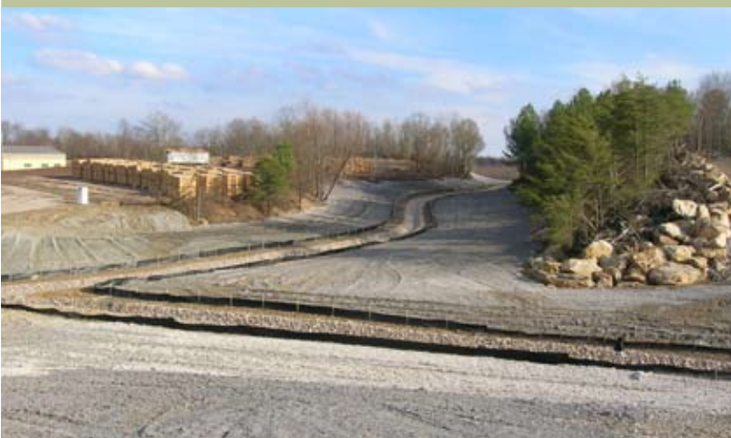
Middleton Run limestone channels Photo by Ian Hughes
