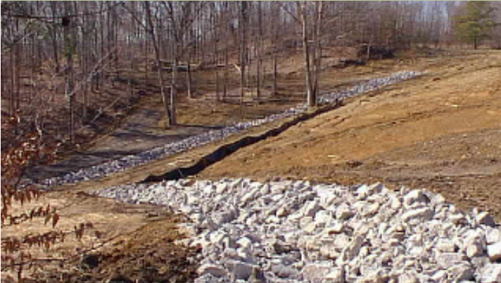
Sr 124 hillside limestone channel, Photo by Chip Rice
