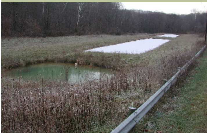
Successive Alkaline Producing System (SAPS), Photo by Ben McCament
