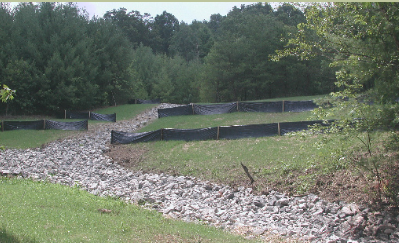
Regraded and resoiled gob pile
