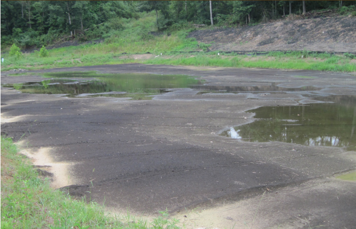
New steel slag bed discharge for Flint Run East at the acid source Photo by Amy Mackey
