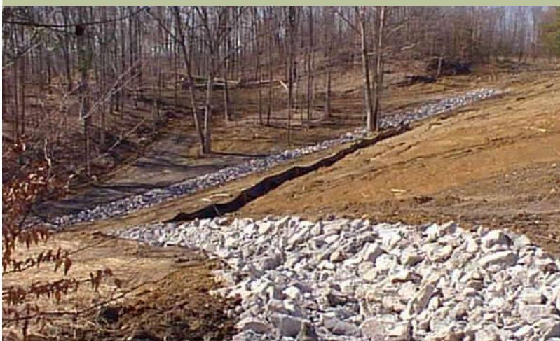
Sr 124 hillside limestone channel Photo by Chip Rice
