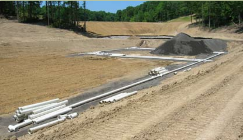
Steel slag bed downstream Lake Milton Photo by Ian Hughes
