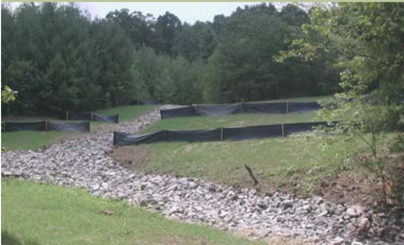
Reggraded and resoiled gob pile Photo by Ben McCament
