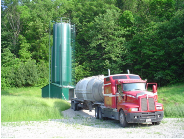
Loading AquaFix Silo
