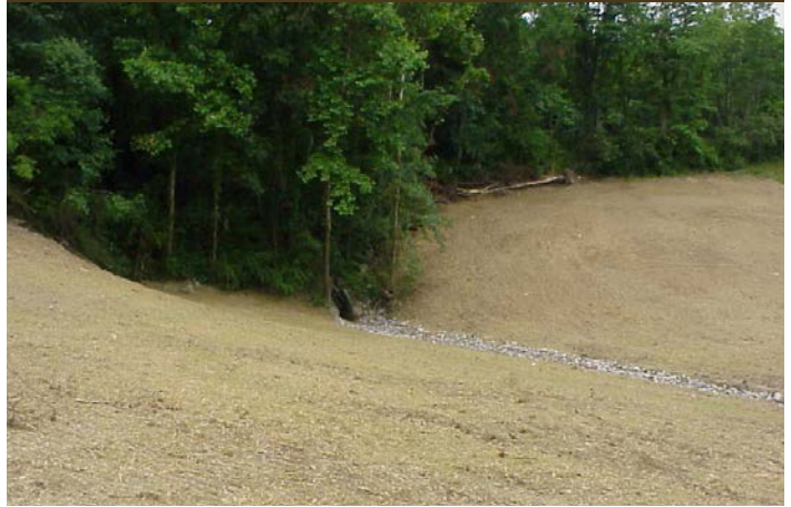
New channel created above old stream capture Photo by Bill Jonard
