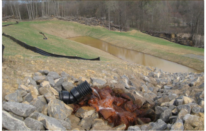
Site two settling pond Photo by Paul Greco
