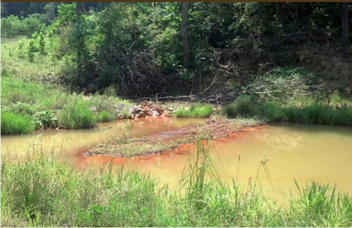
Lyons II limestone berm in settling pond
