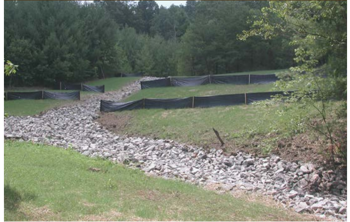
Regraded and resoiled gob pile Photo by Ben McCament
