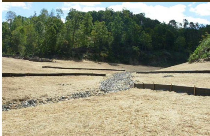
West Branch Sunday Creek Phase I post reclamation featuring a limestone channel. Photo by Sunday Creek Watershed Group
