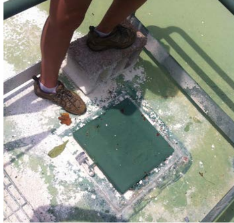
New manhole installed on top of Jobs Hollow Doser Photo by Nate Schlater
