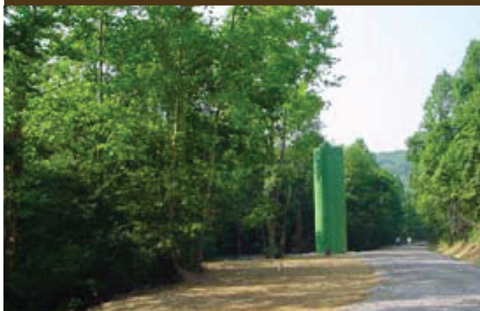
Jobs Hollow Doser Photo by Monday Creek Restoration Project
