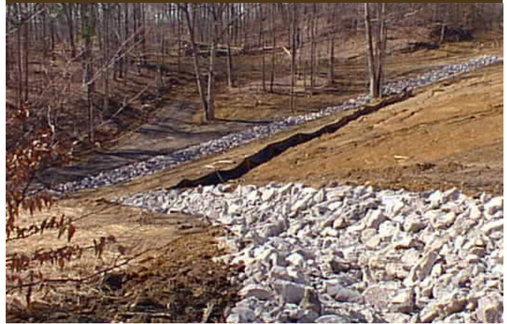
Sr 124 hillside limestone channel Photo by Chip Rice
