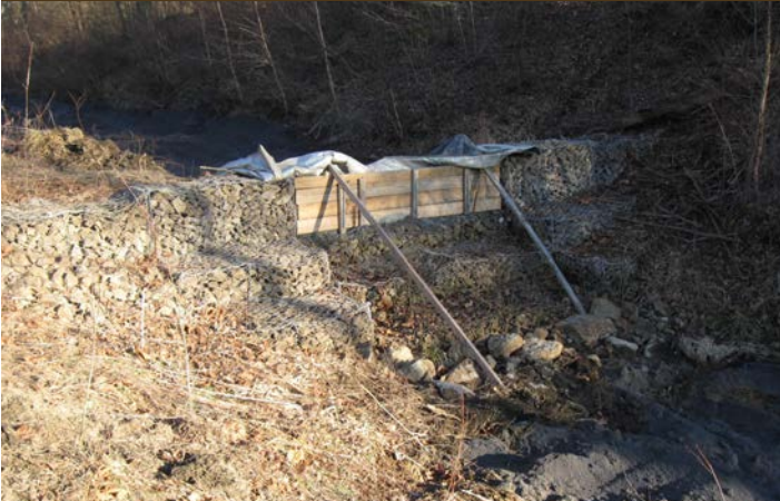
EB Phase I site 8 slag bed Photographer: Amy Mackey
