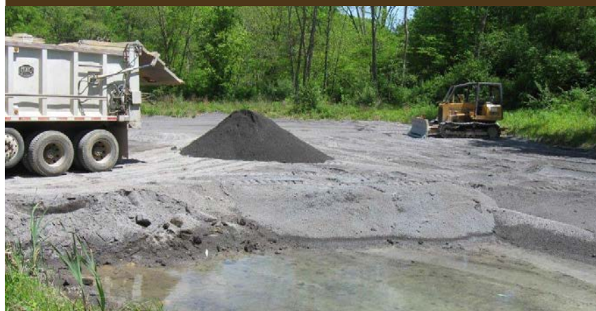
New slag being added to the Lost Run slag bed Photo by Nate Schlater
