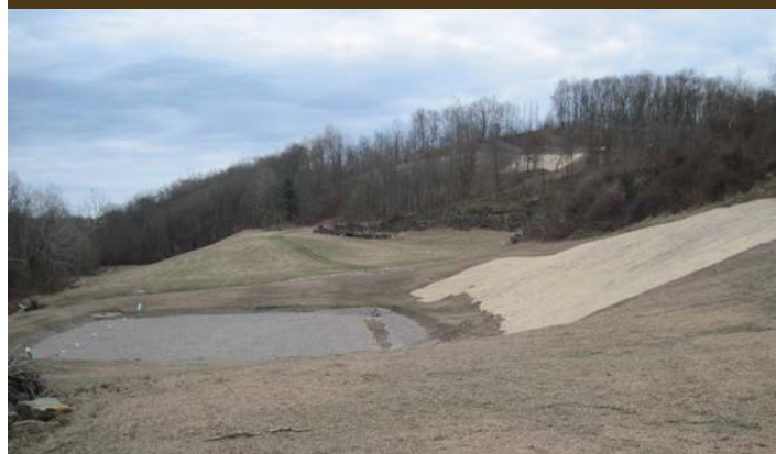
West Branch Headwaters limestone leach bed. Photo by Michelle Shaw
