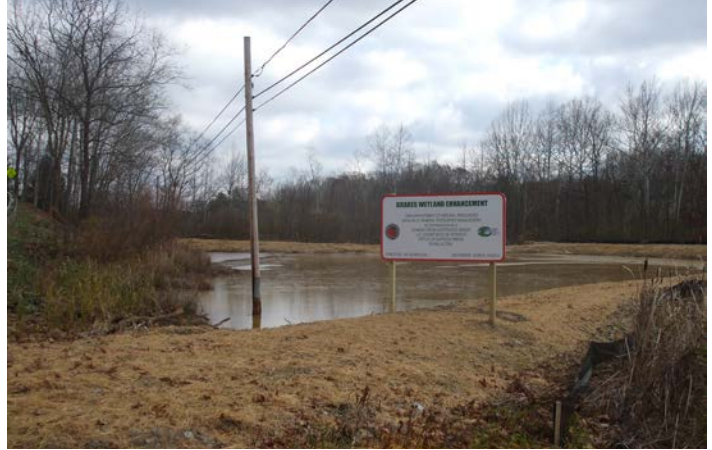
Drakes Wetland Enhancement Completion sign Photo by Mike Gosnell
