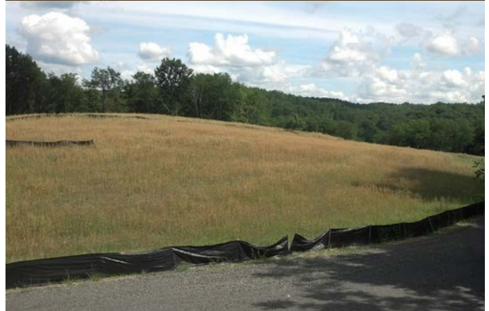
Hilltop Energy post-construction Photo by Huff Run Watershed Group
