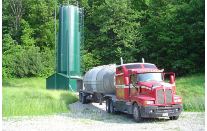
Carbondale II Project Doser Photo by JT Kneen
