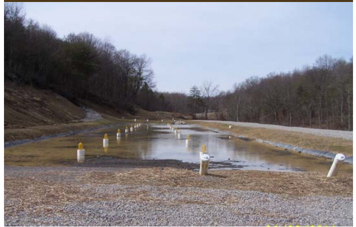
Steel slag bed at Kern Hollow Photo by Amy Mackey
