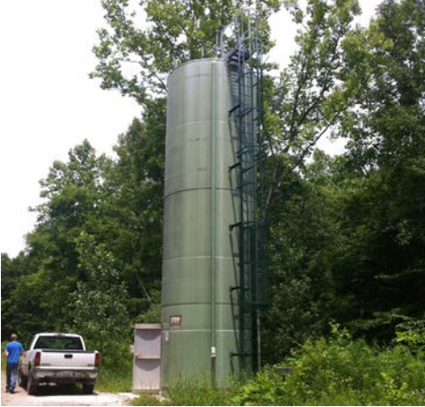
New ladder installed on Jobs Hollow Doser Photo by Nate Schlater
