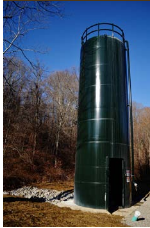
Pine Run Doser post-construction photo Photo by Sunday Creek Watershed Group
