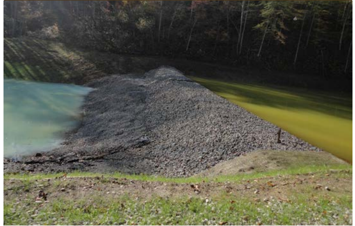
Coe Hollow Limestone Leach Berms (USFS) Photo by Monday Creek Restoration Project
