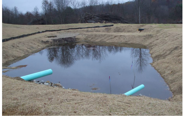
Sludge precipitation basin downstream of limestone leach bed Photo by Frank Martin
